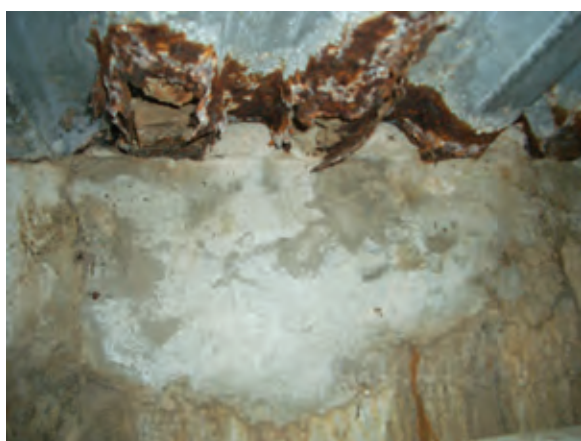
Figure 1-4 Corrosion of galvanized fluted steel floor deck. The floor is at grade level. The source of the water is rainwater seepage.
