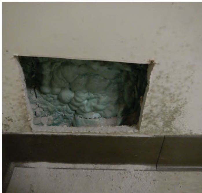
Figure 4-1 Interior Wall Showing Water Damage and Mold
